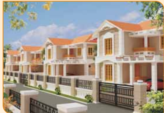
NANDANAM PARADISE VILLAS Thrissur
